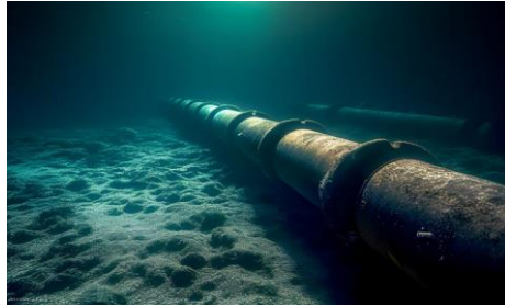
Inspection of installations
